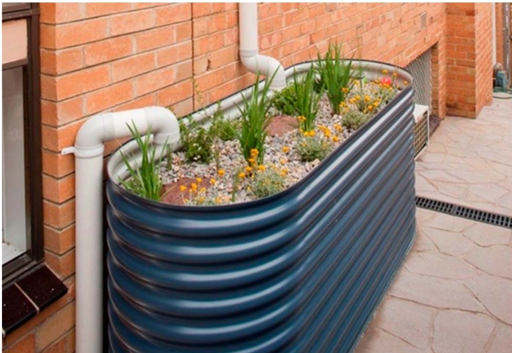
Figure 9: Above-ground raingarden planter (source: Melbourne Water)
